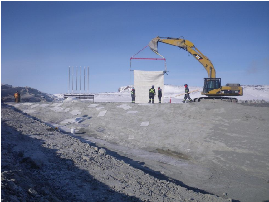
Photo 5: Placement of upper GC south of station 0+50.
