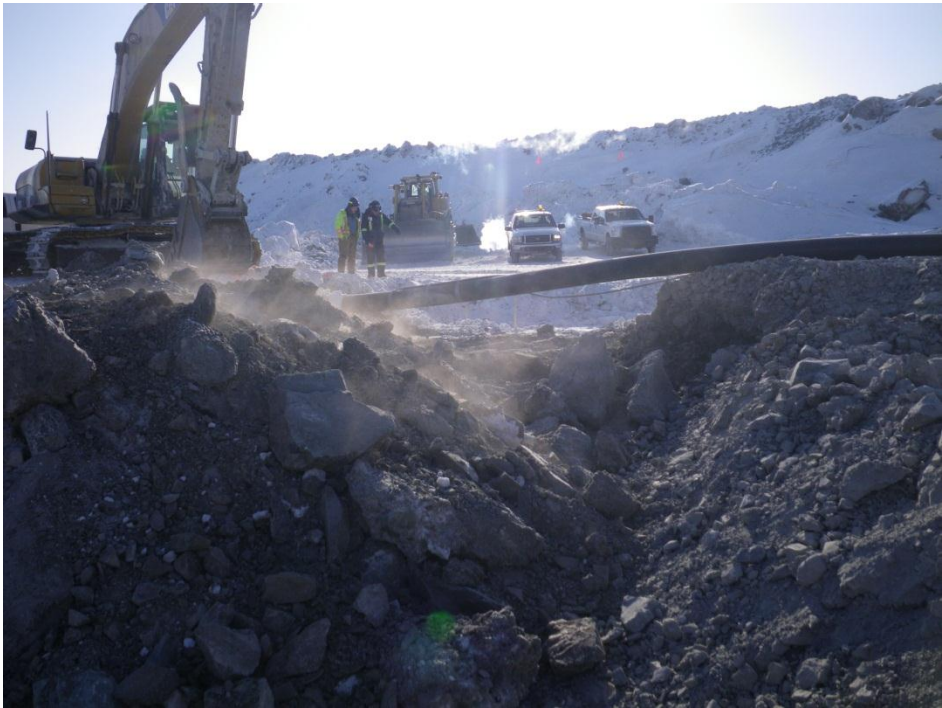
Photo 6: Diversion Berm - Excavation through primary road for culvert installation.
