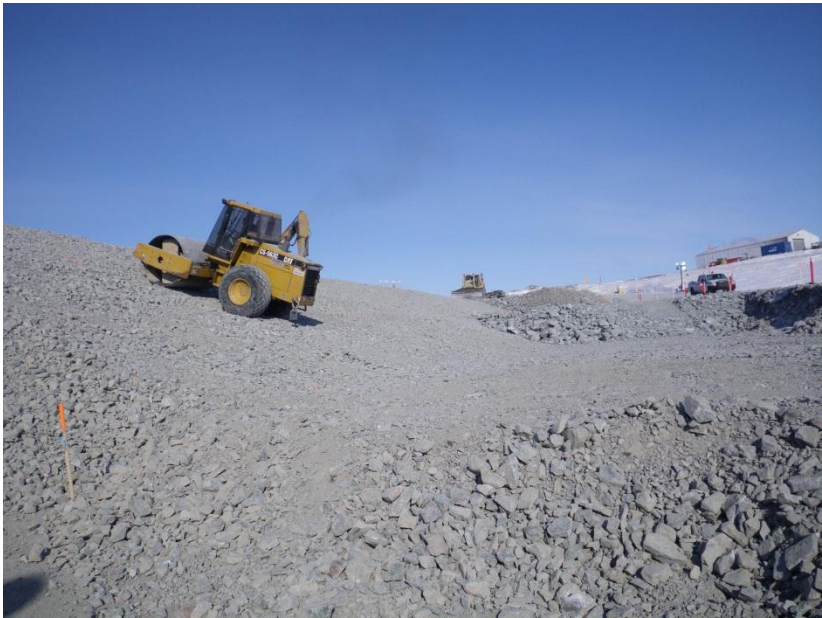
Photo 9: North Dam - Compactor compacting slope of transition material. Photo looking north east along dam alignment.
