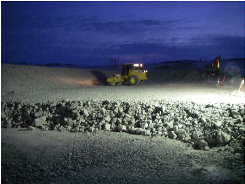
Photo 11: Compactor on the first lift of ROQ on the upstream side.
