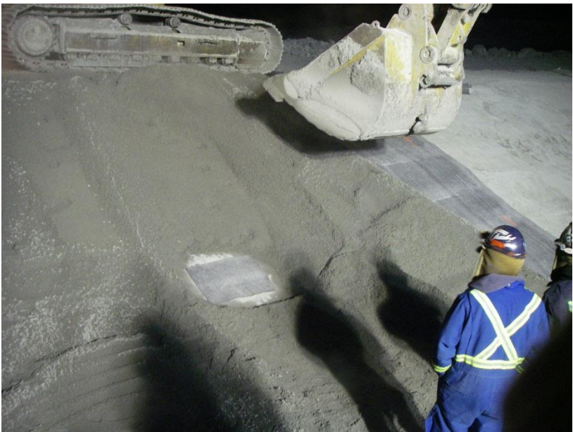
Photo 10: Patch in the GCL liner.
