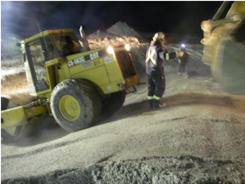
Photo 11: Compactor on the first lift of ROQ on the upstream side.
