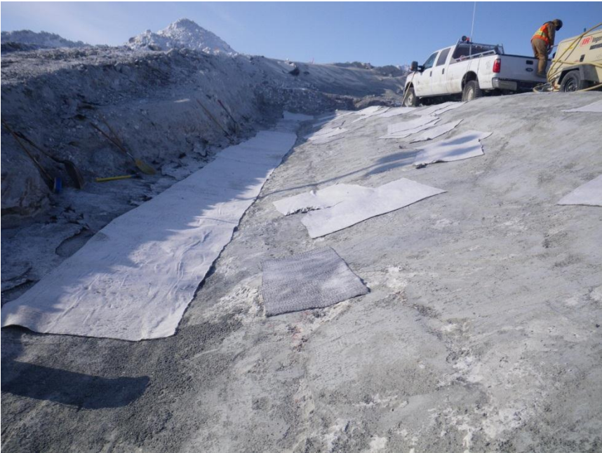
Photo 4: large patches placed over the GCL liner south west of station 0+50.
