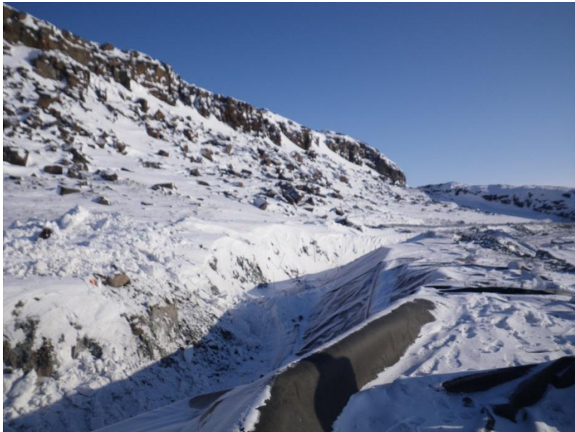
Photo 8: View of the diversion berm where snow was allowed to accumulate on the exposed geotextile and HDPE liner.
