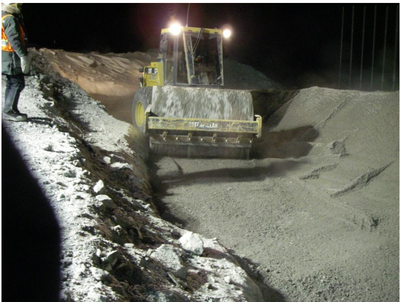
Photo 12: Compactor compacting the toe of the overliner material. Photo looking south.
